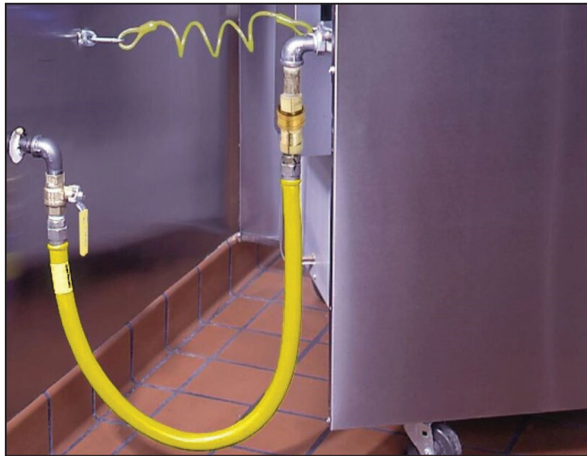
APPLIANCE CONNECTOR INSTALLED
