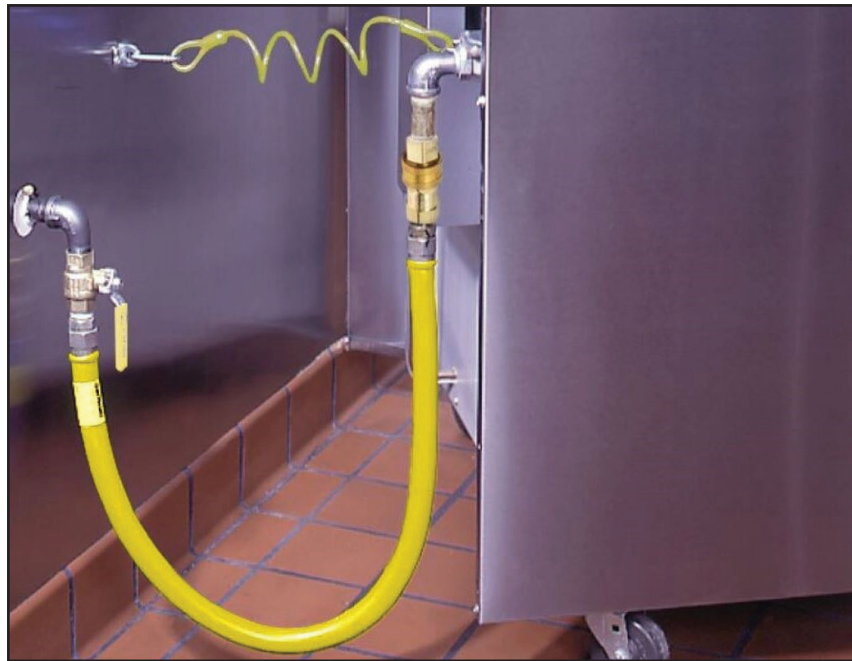
APPLIANCE CONNECTOR INSTALLED
