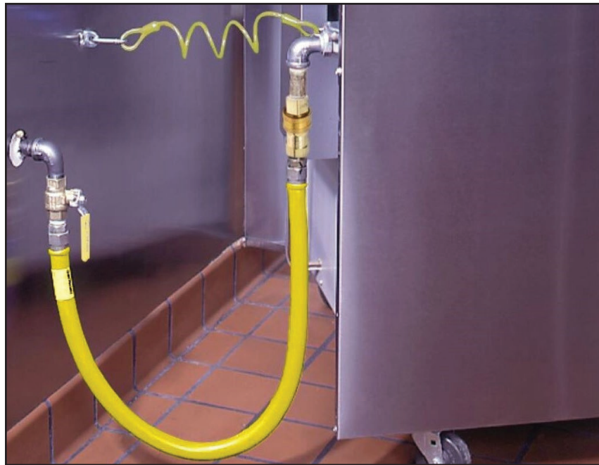
APPLIANCE CONNECTOR INSTALLED
